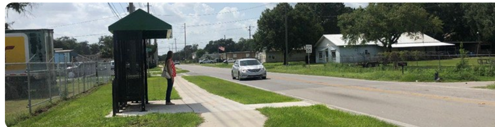
Citrus Connection Bus Shelter
